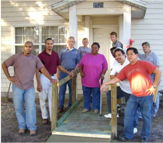
CIL volunteers helped build this wheelchair ramp.
